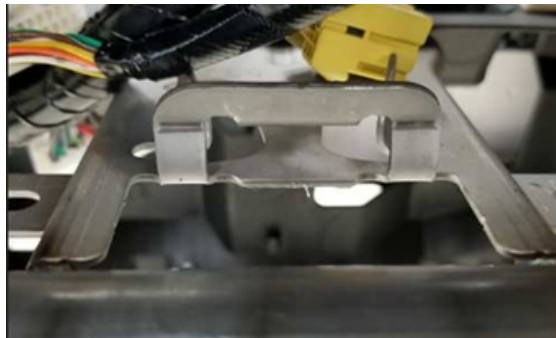
Bend up factory metal bracket on dash bar to allow clearance for brace bar clamp.
